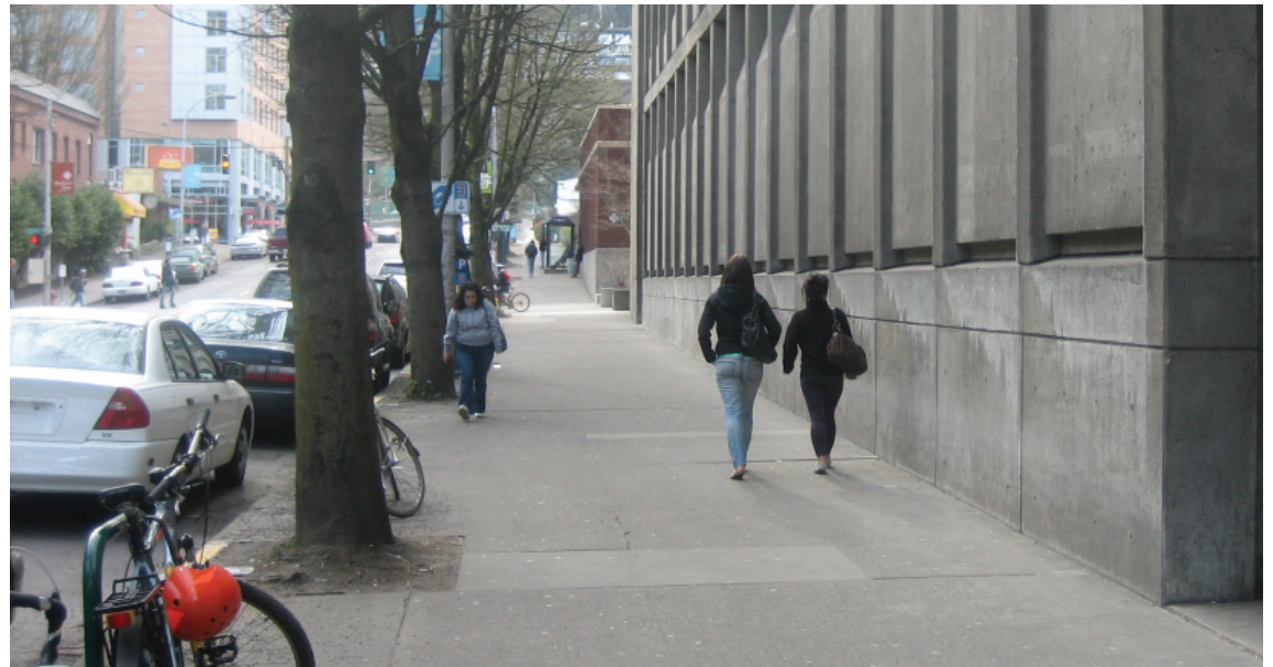
Neuberger Hall Facade along SW Broadway
