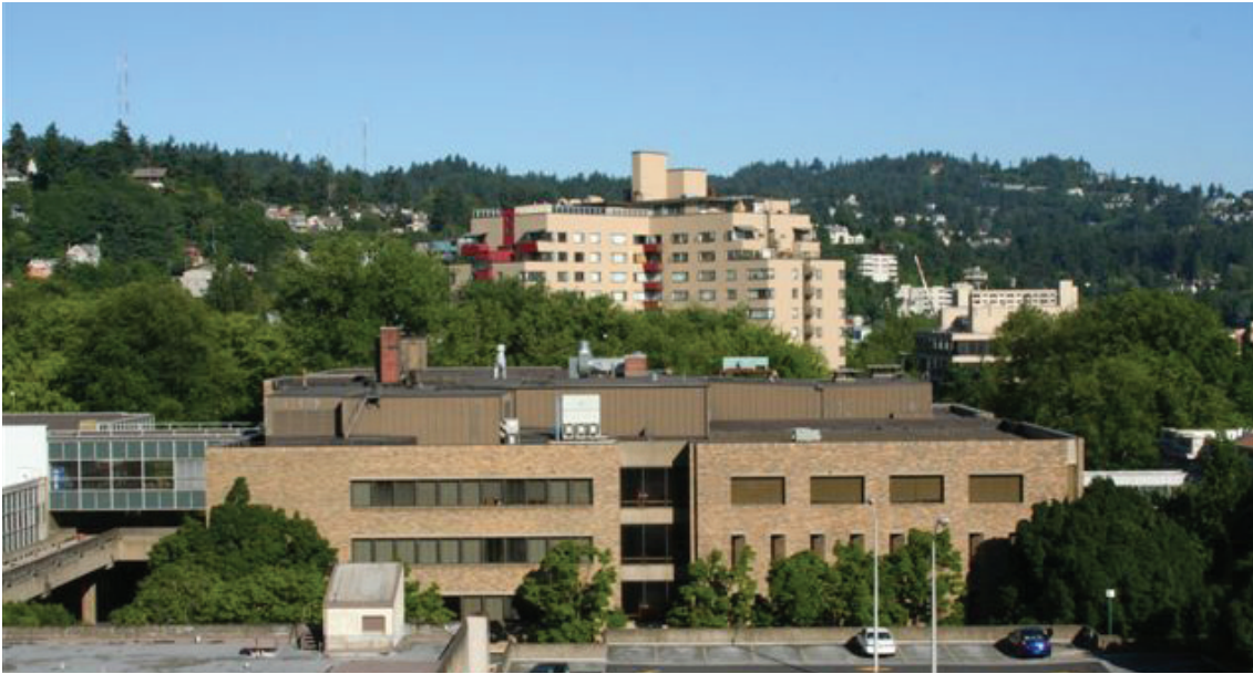
View of Cramer Hall
