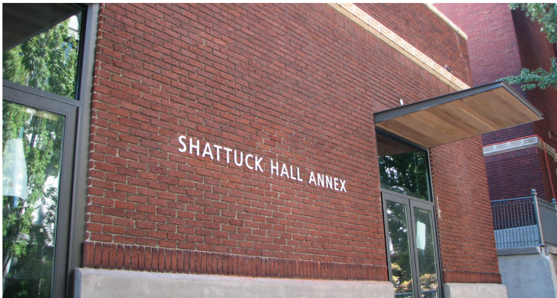
Renovations of the Shattuck Hall Annex
