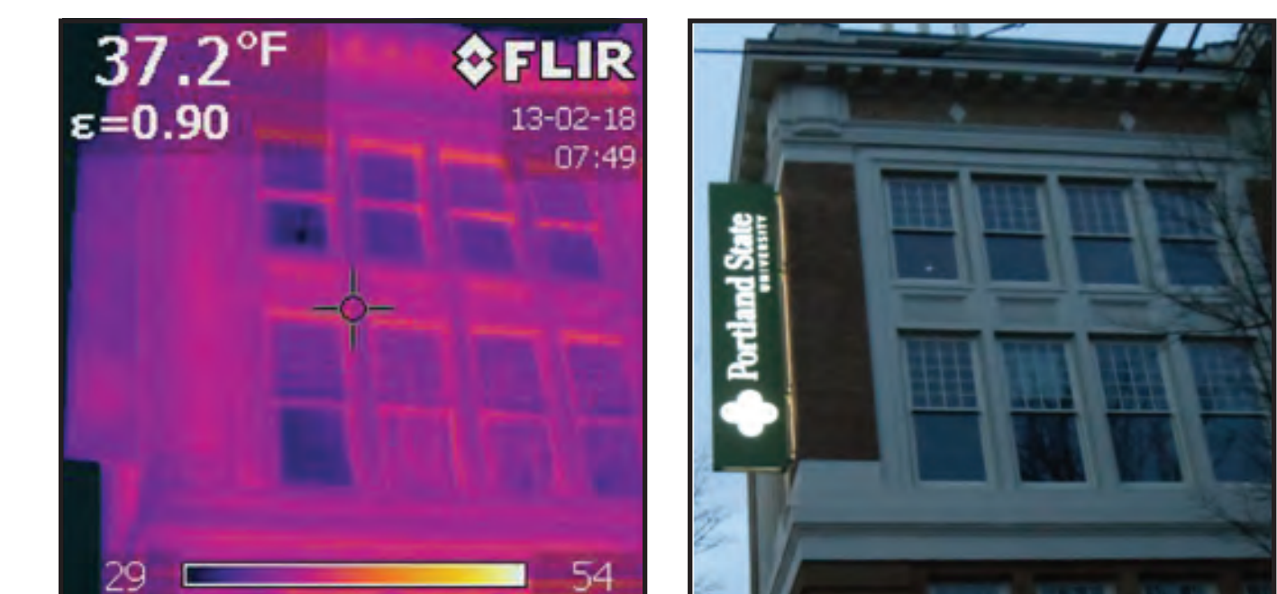
Figure 2.3 - Lincoln Hall post-retrofit 2010. has a highly efficient envelope, with a surface temperature equal to the ambient outdoor air.
