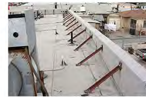
Roof Parapet Bracing
