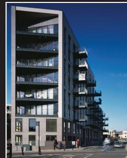
Project: Bridport House Location: Hackney (London), UK Architect: Karakusevic Carson Architects Completed 2011 Description: 8 story Residential Construction: Platform-based CLT system
