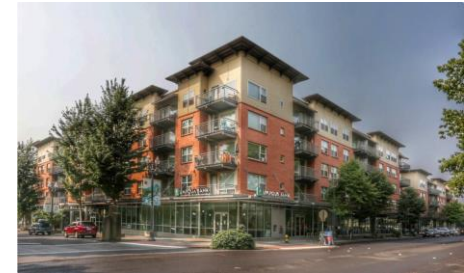
Esther Short Commons - 2004 Vancouver Housing Authority 160 Units
