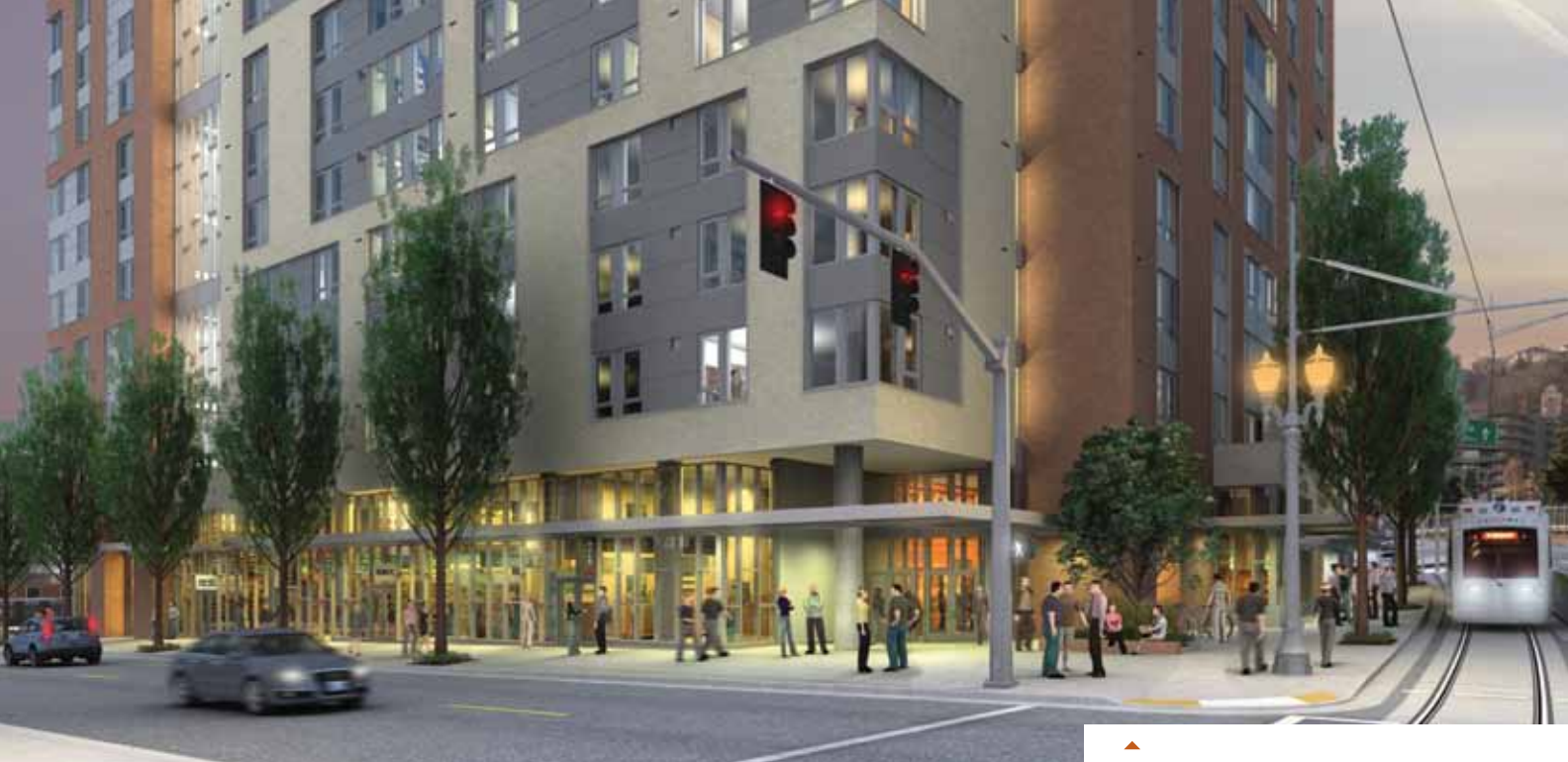
▲ University Pointe, PSU's newest residence Hall, is being built with $90 million in private money.
