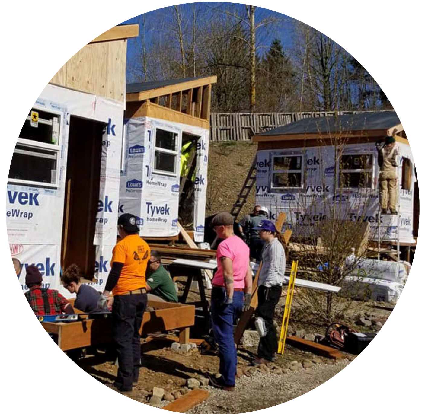
Volunteers and Cascadia Clusters building pods Image credit: Agape Village
