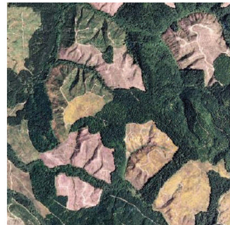
Aerial photo, South of Vernonia, OR
