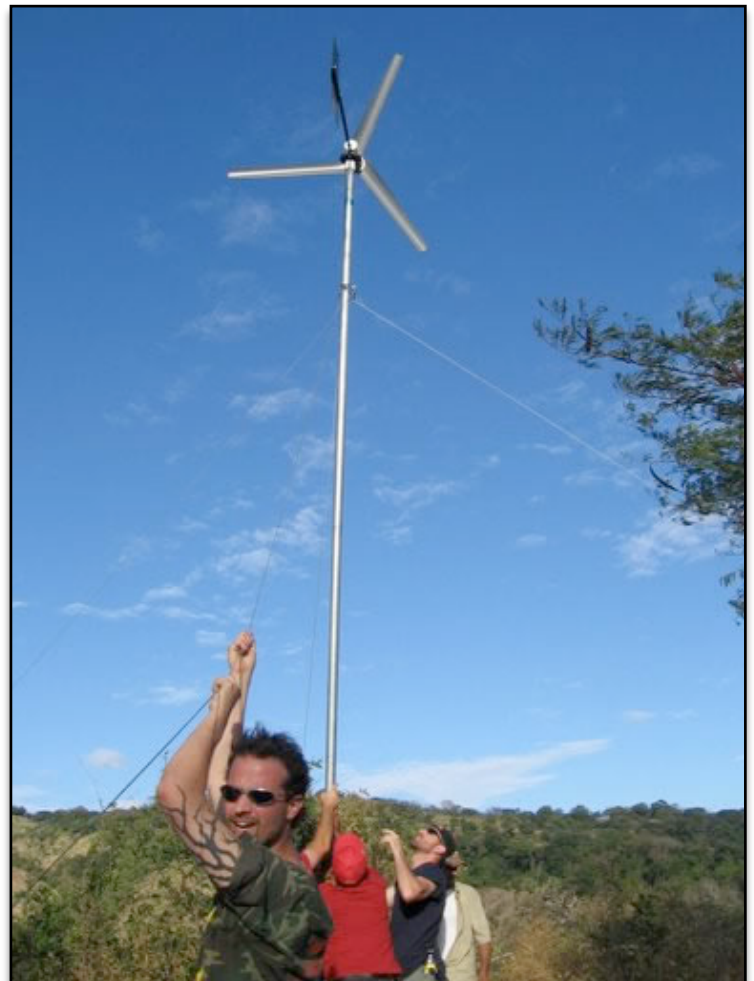
ESM alumnus Greg Price (front) installing a wind turbine.
