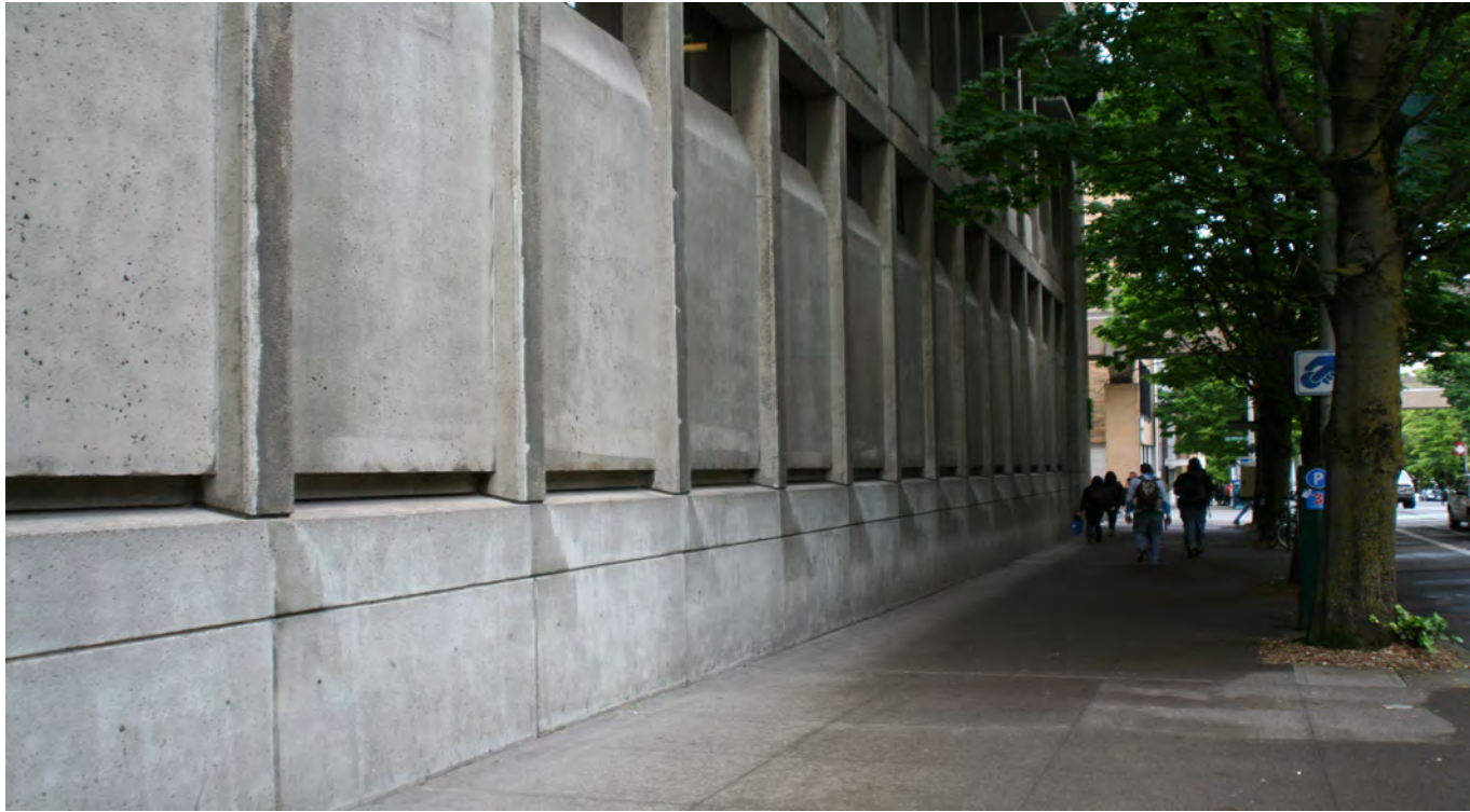
Figure 7 Existing Broadway Ground Floor Facade
