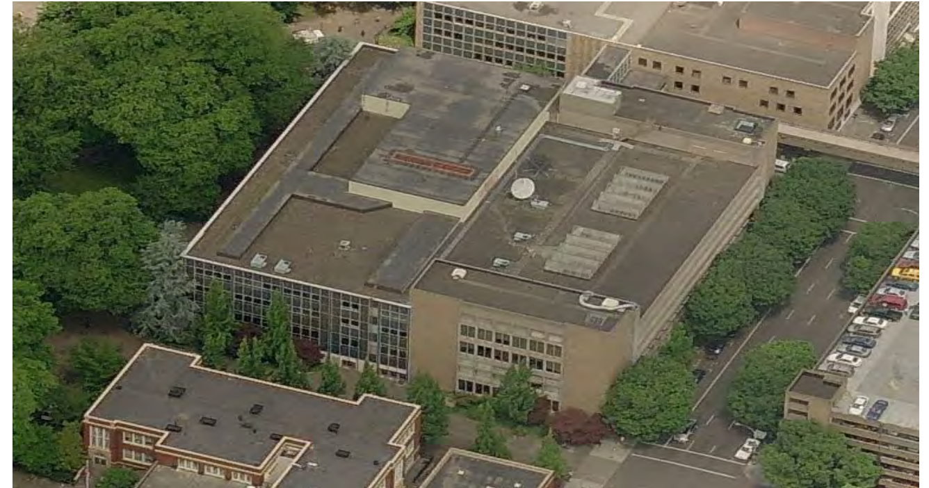
Figure 14 Neuberger Hall Roof From Southeast
