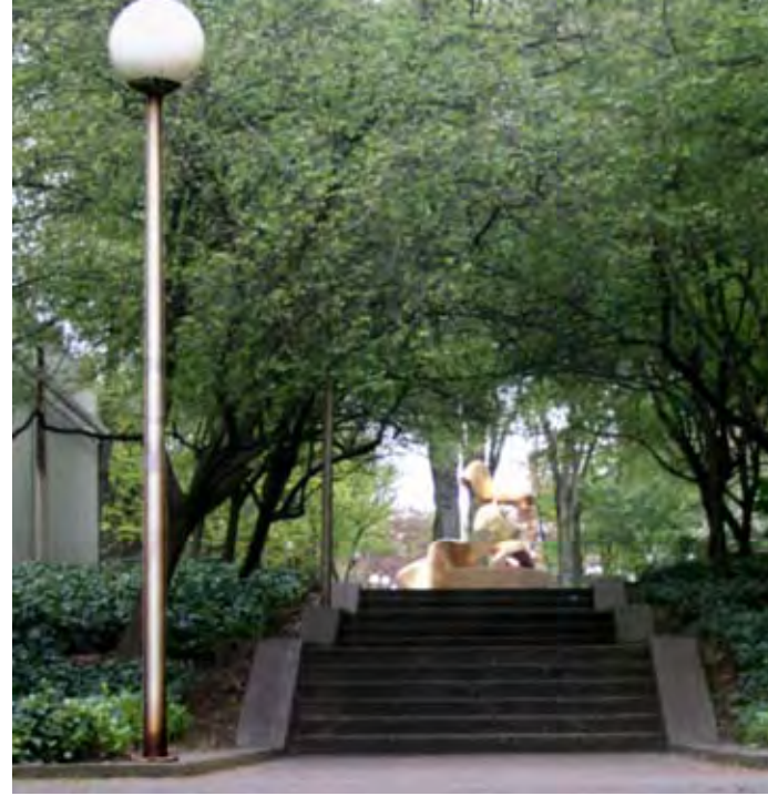
Many of the existing light poles are in need of restoration.
