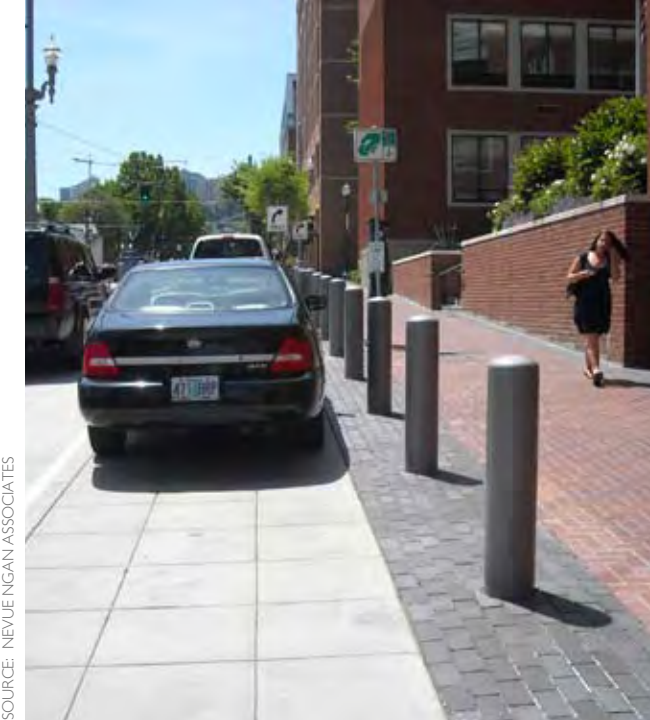
Bollards separate the sidewalk from the parking zone along this curbsless street.
