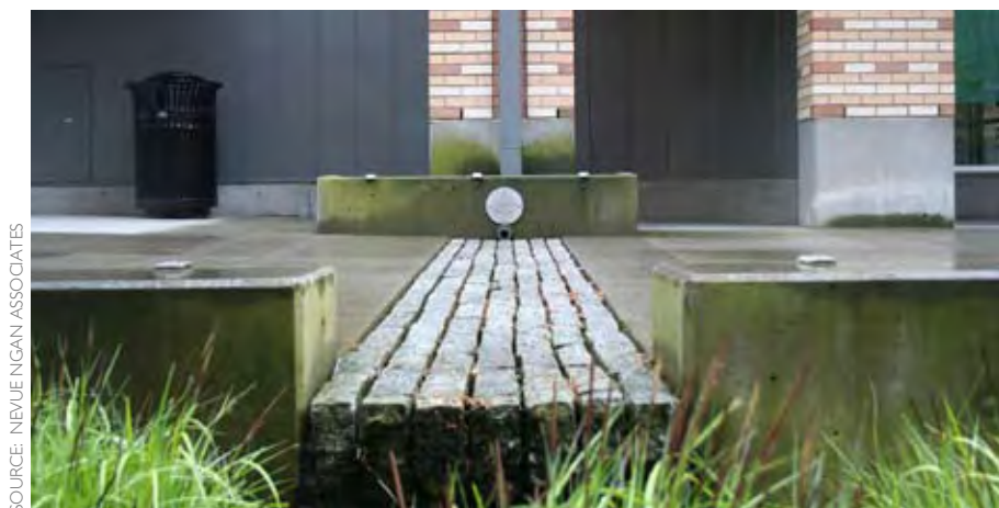
The stormwater planters along SW Montgomery and Epler Hall recycles rainwater back into the building for reuse.
