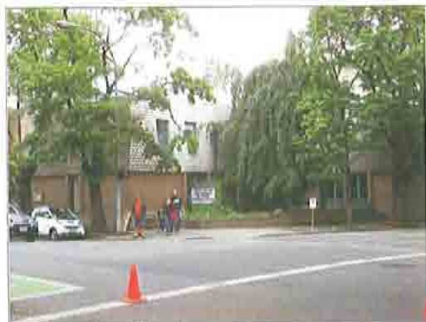
South and west facades
