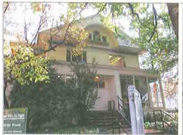
Front (west) façade
