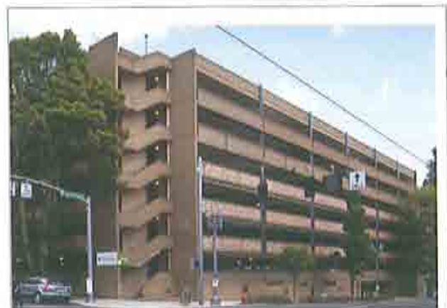
South and west facades
