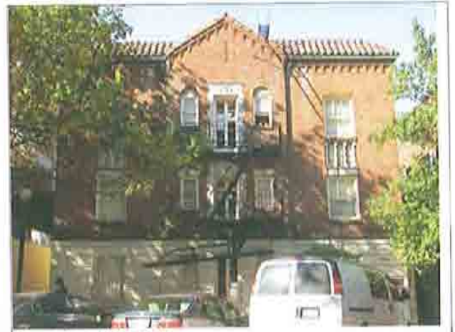
Front (east) façade
