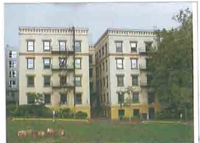
Front (east) façade
