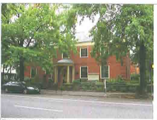
Front (east) façade
