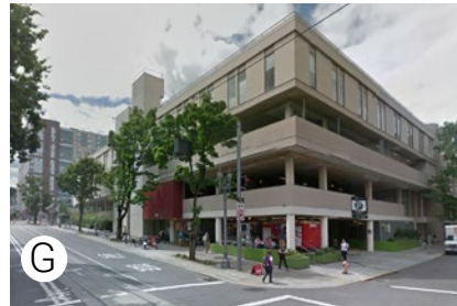
University Center Building Stories: 4 stories, Program: Education, Health
