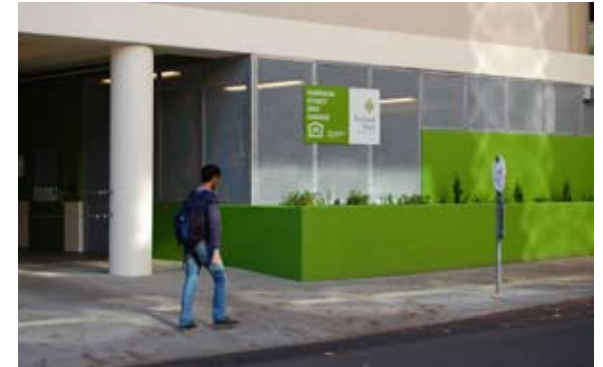
The Harrison Street Bicycle Garage is accessible through a ground-level entrance on the north side of University Center Building and has been made more visible and prominent through signage and streetscape improvements along this busy stretch of Harrison Street.
