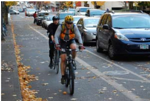
The Broadway Cycletrack, an at-grade bicycle route separated from traffic by an automobile parking lane, runs southbound through campus from SW Clay to SW Jackson.
