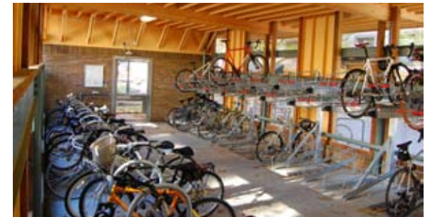
Seventy-seven bicycles can lock up to the Montgomery Street Bicycle Garage on a range of articulated and staple racks. A key-card access control entry door to the structure and closed-circuit cameras help ensure the security of bicycles in the facility.
