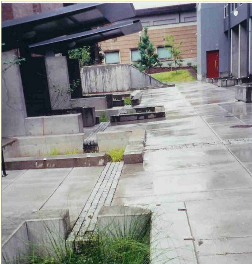
Figure 2: Stormwater planters drain to rainwater storage tank below the plaza (5/2004)
